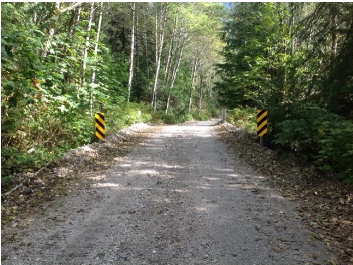
Approach from Right Bank when facing downstream
