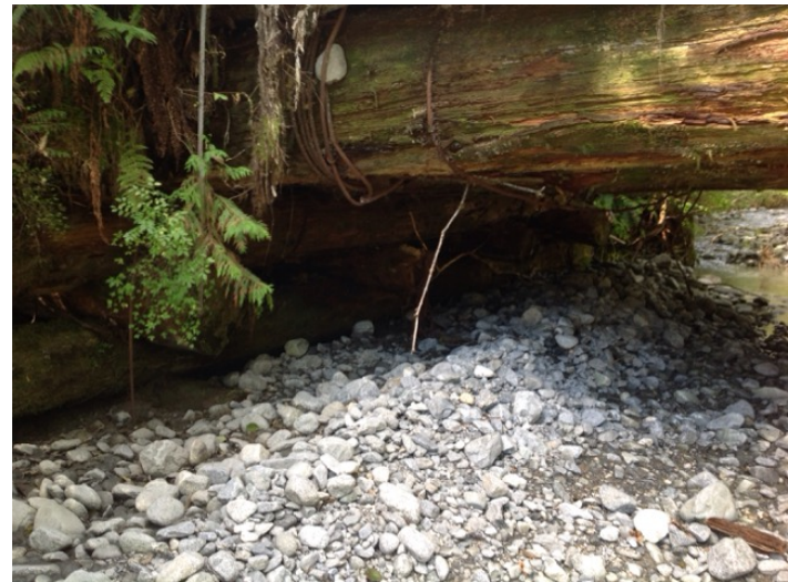
Right Bank Abutment when facing downstream
