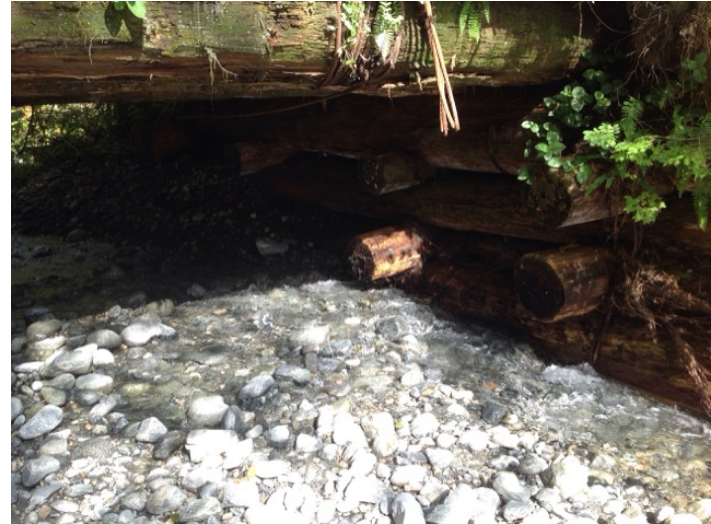
Left Bank Abutment when facing downstream
